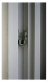
Using a regular straight screwdriver, turn the metal cam in the pivot shoe so the cam slot is horizontal or in the unlocked position. Using the screwdriver, position the left side 3 inches above the top of the sill and rotate the cam so the cam opening is at the top. This activates the brake and the shoe will remain in this position. Repeat on right side.
